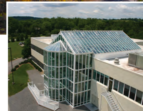
Constructed in 2005, this aluminum and steel reinforced PVC conservatory encloses a former parking area and is now a showroom space.
