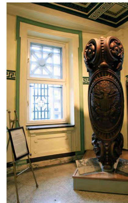
Original wood double hung window replaced by a vinyl tilt-turn over tilt-turn
