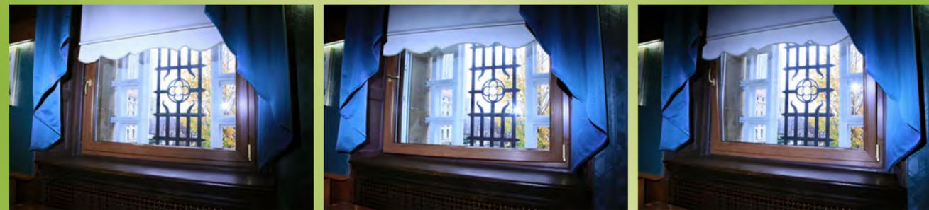
Golden Oak woodgrain laminate tilt-turns were chosen to match the original hungs. Shown (left to right) in closed position, turn position for easy cleaning and tilt position for ventilation
