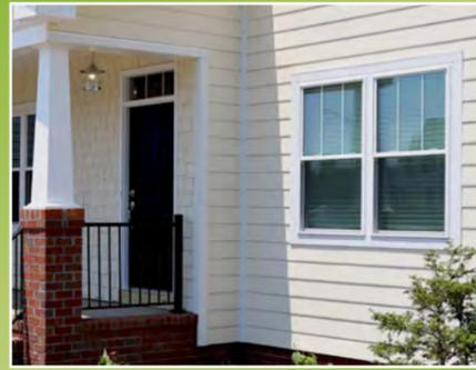
Two mullied double hung windows allow for more light to enter the home while minimizing visual obstruction and using less framing material during installation.
