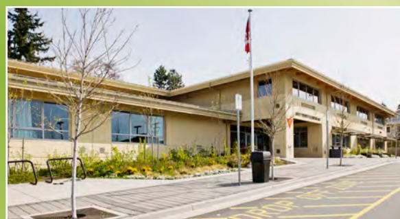
Contemporary aluminum look painted PVC frame and sash provides significantly improved thermal performance.
