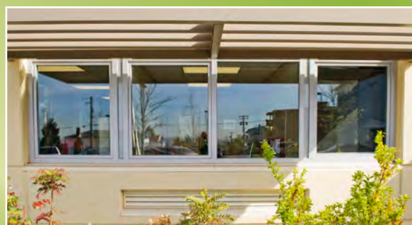
Contemporary aluminum look painted PVC frame and sash provides significantly improved thermal performance.
