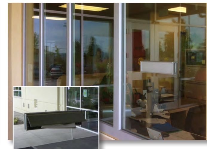
Cut in mail slot to center of sealed unit in office area solved problem as no other convenient space to install mail slot.
